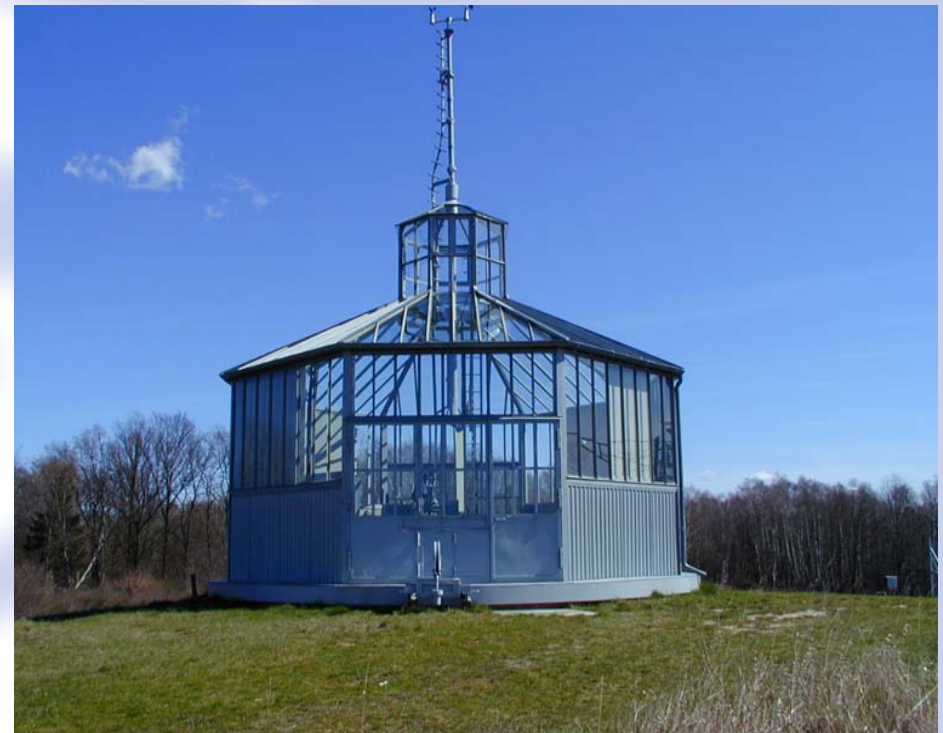
The winch house at Lindenberg Observatory : Technical monument for the operational monitoring of atmospheric parameters using kites in the last century
