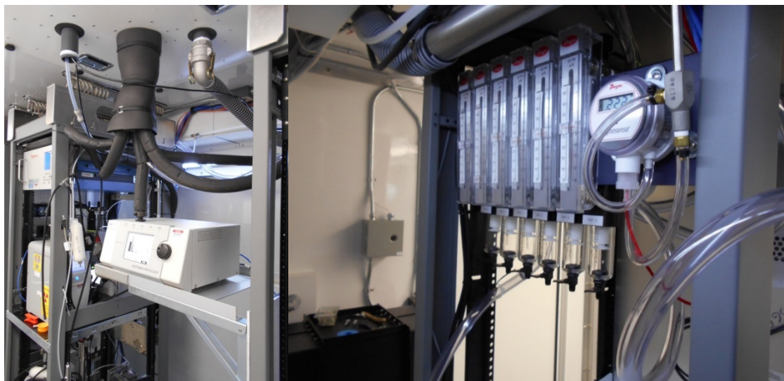
Figure 8. AOS07 flow distributor and bypass manifold.
