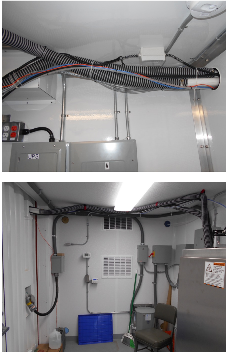
Figure 6. AOS07 cable pass-through opening and interior view of the cable bundle.
