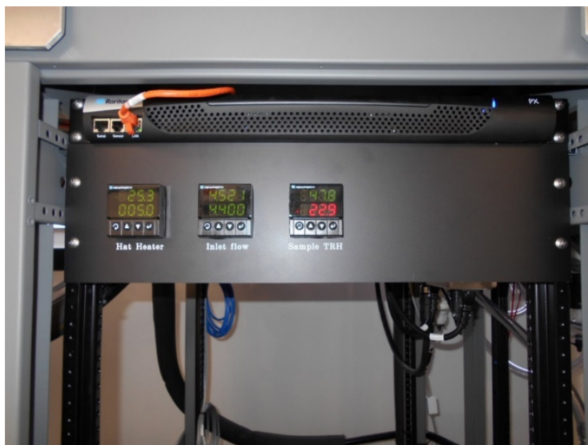
Figure 9. AOS07 monitoring console.
