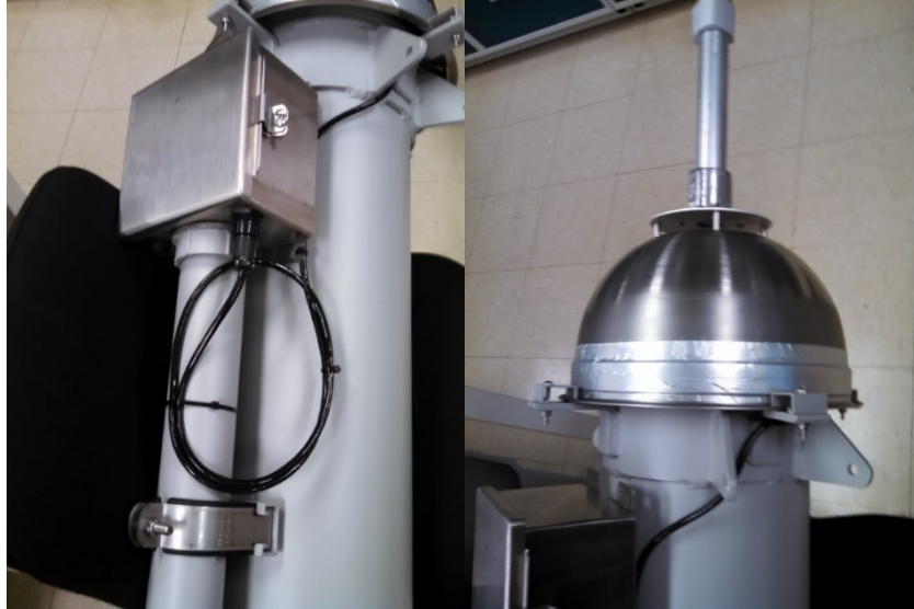
Figure 3. The junction box and the rain hat at the top of the aerosol inlet.
