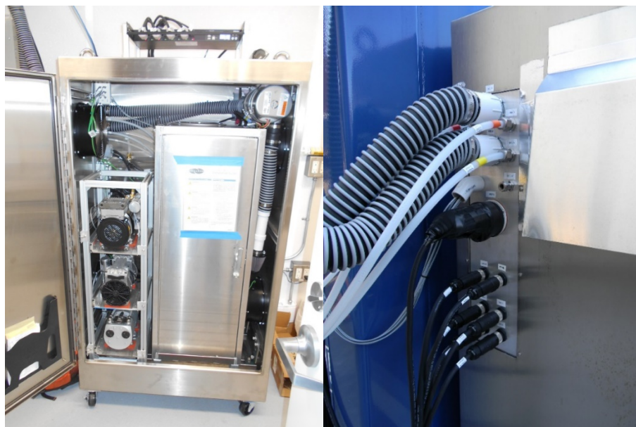
Figure 5. AOS07 blower enclosure interior and connection panel.
