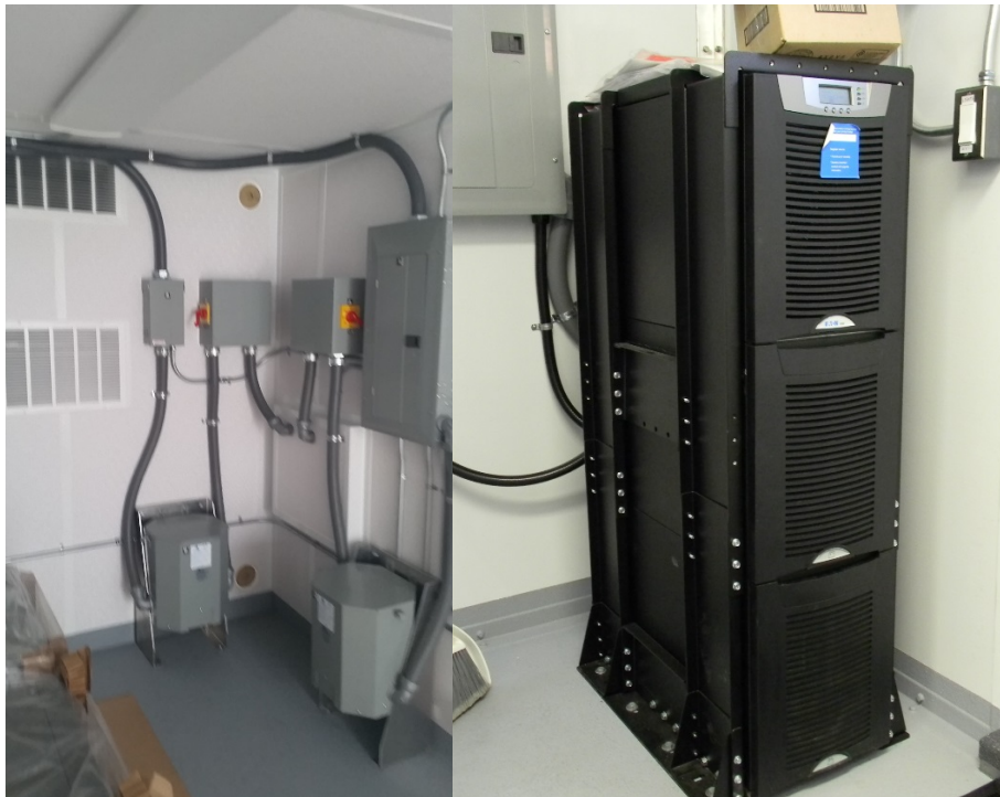
Figure 11. AOS07 power main panel and UPS.
