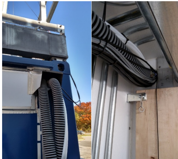
Figure 6. AOS03 cable pass-through opening and interior view of the cable bundle.
