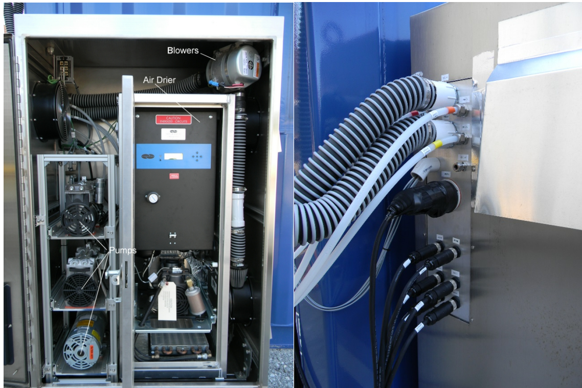
Figure 5. AOS03 blower enclosure interior and connection panel.
