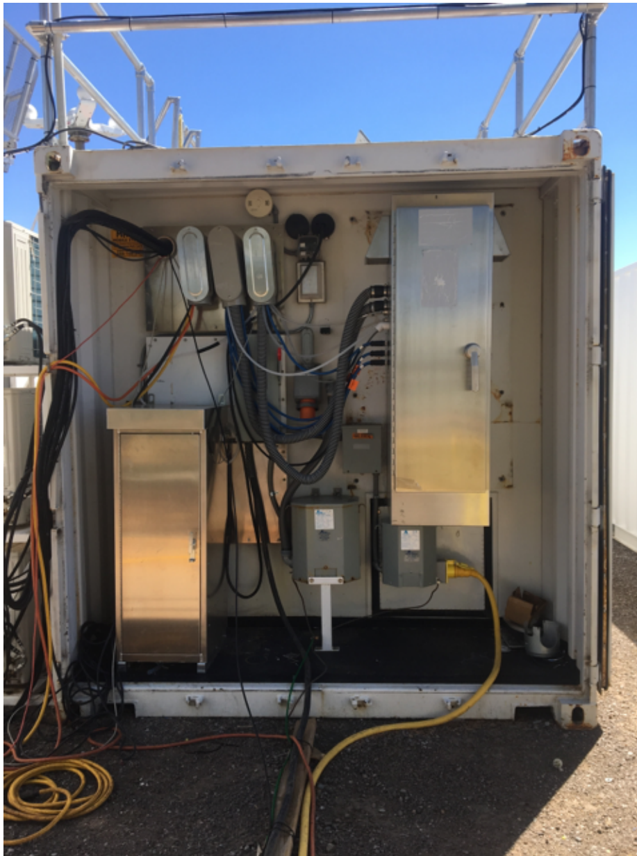
Figure 4. The rear vestibule of the AMF2 AOS (AOS02): (left) air dryer; (right) pump enclosure; (bottom middle) power transformers.
