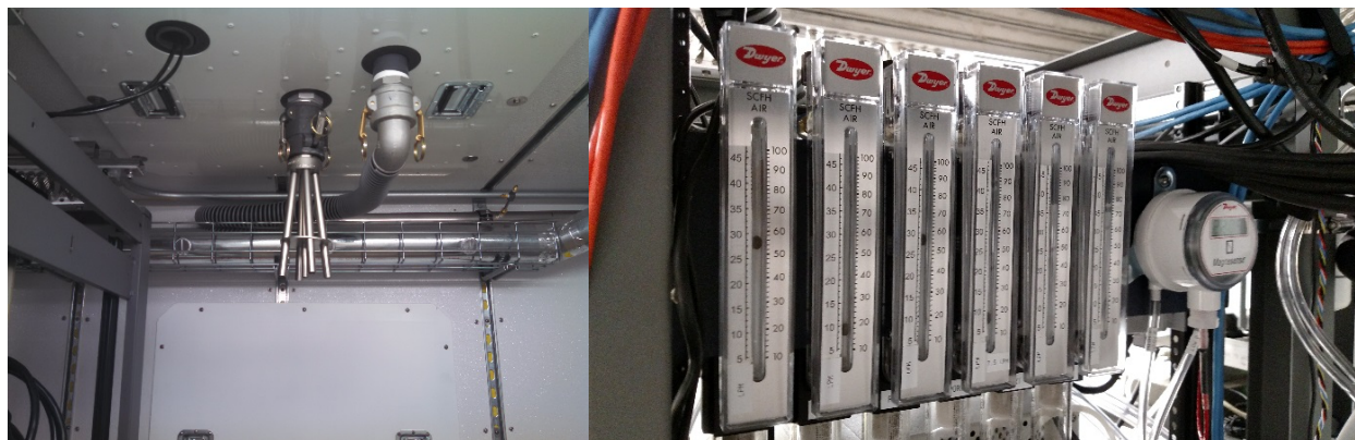
Figure 7. AOS02 flow distributor and bypass manifold.
