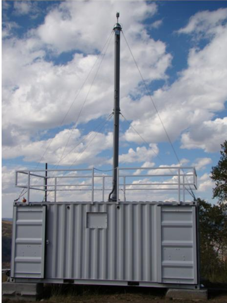
Figure 6. Aerosol Observing System (AOS) instrument enclosure with 10 m sampling stack.
