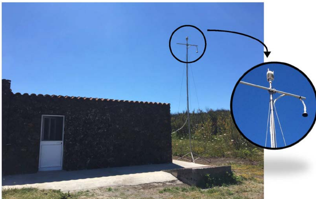
Figure 2. S1 with the aerosol inlet and Meteorology sensor located at \sim 3 meters above the roofline.
