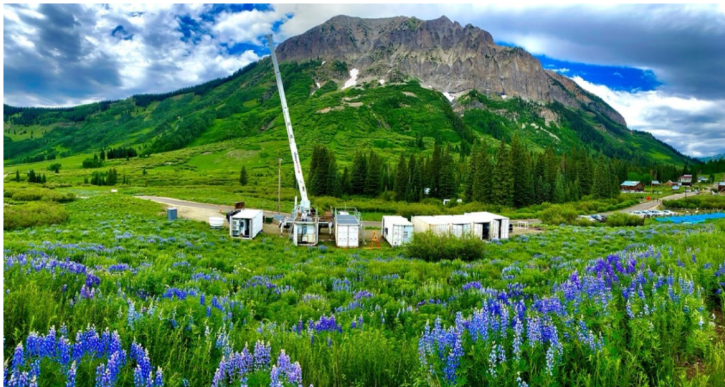
Figure 5. Containerized instruments of the AMF2 at the SAIL M-1 site at the base of Gothic Mountain during the installation phase of SAIL. Photo taken by Ken Williams in June, 2021.
