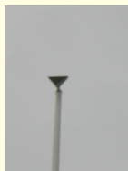
New tower mounted WACR corner reflector.
