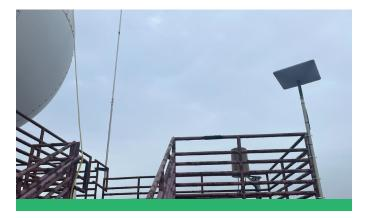
A Starlink system is shown at ARM's North Slope of Alaska atmospheric observatory.
