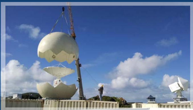
The final large instrument to be installed at the ENA observatory, the X-band scanning ARM precipitation radar (X-SAPR) operates in a simultaneous transmit and receive mode, meaning that the transmit signal is split so that power is transmitted on both horizontal and vertical polarizations at the same time.
