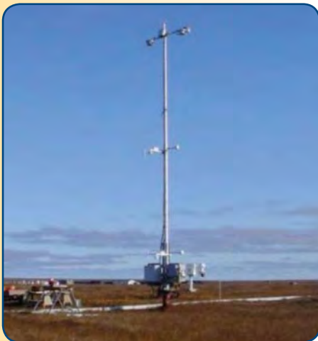
Met towers at the ACRF Barrow and Atqasuk (shown here) sites are sporting new instrumentation that improves data delivery and requires less maintenance.
