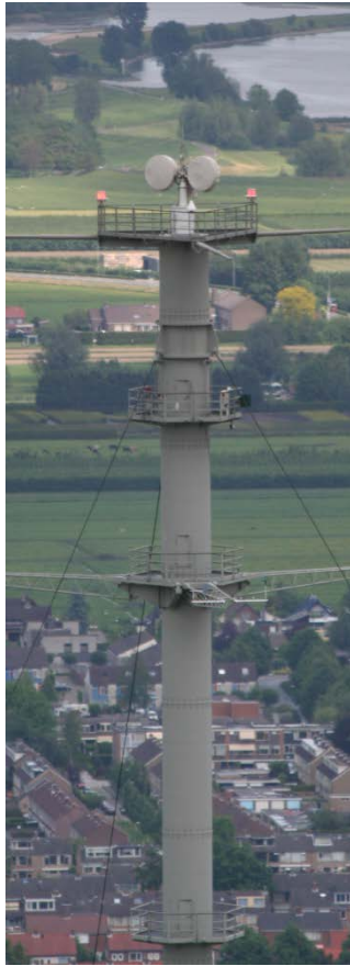
IDRA is mounted on top of the 213 m high meteorological tower.
