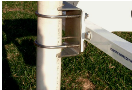
Figure 2.1 Installing Mounting Bracket & U-Bolts
