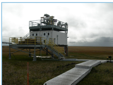
North Slope of Alaska
