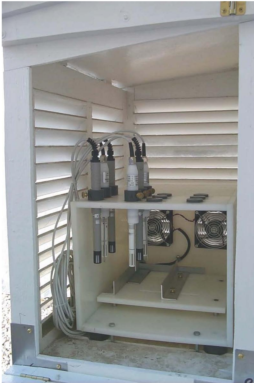
Figure 4. The new system for surface meteorological reference measurements to be installed at the SPG radiosonde launch site. The inner chamber houses 6 T/RH sensors, ventilation fans, and a switch that records when a radiosonde is placed upon it. The outer “Stevenson screen” shelters the sensors from solar heating and rain.
