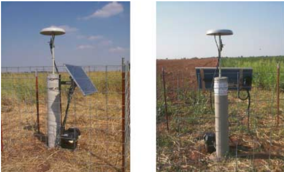
Figure 2. Two L1 GPS systems are shown. Each system consists of a GPS receiver, a radio modem, and has solar power with battery backup.
