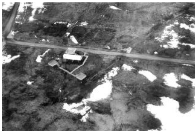
Figure 1. Aerial view of the instrument shelter and associated instrumentation decks at the NSA/AAO Barrow facility before any instrumentation was mounted. The 40-m meteorological tower is just above the upper boundary of the photograph.
