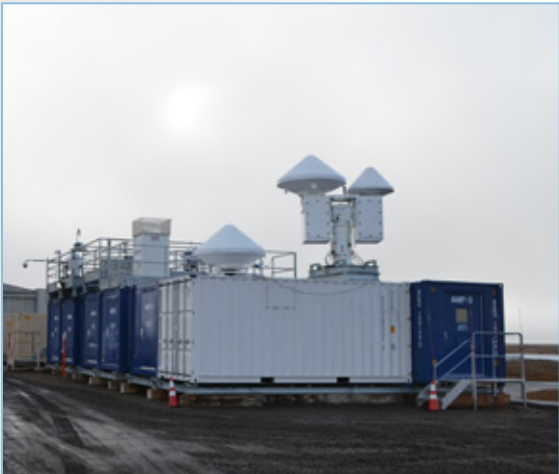
The second phase of the third ARM Mobile Facility installation will be completed in the fall of 2014 with the addition of scanning and vertical-pointing radars, as well as a Raman lidar.
