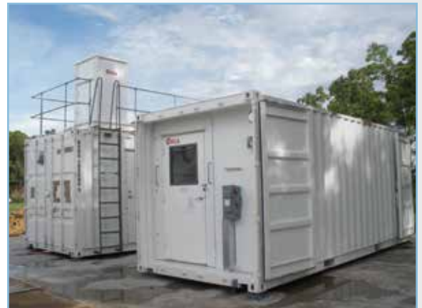
The Darwin site's new Raman lidar (in rear) is housed in a climate-controlled 8'x8'x20' standard shipping container. An additional shelter (in front) houses the water chiller, power supply, and electrical distribution systems that support the lidar.
